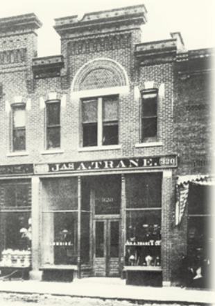
Trane Storefront La Crosse, Wisconsin 1891
