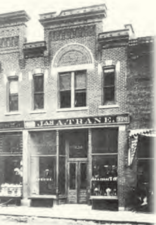
Trane Storefront La Crosse, Wisconsin 1891
